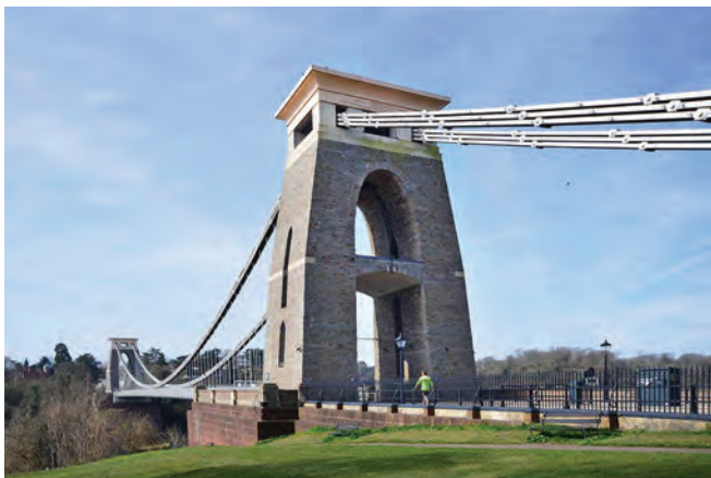
Clifton east abutment tower in foreground with the west Leigh Woods abutment beyond at the far end of the bridge
